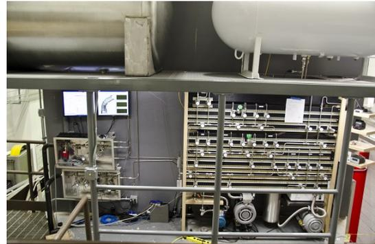
**Figure 8.38:** (Color online) Methane and deuterium gas handling systems.
